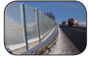
NOISE PROTECTION WALL SECURED FROM BIRD COLLISIONS
